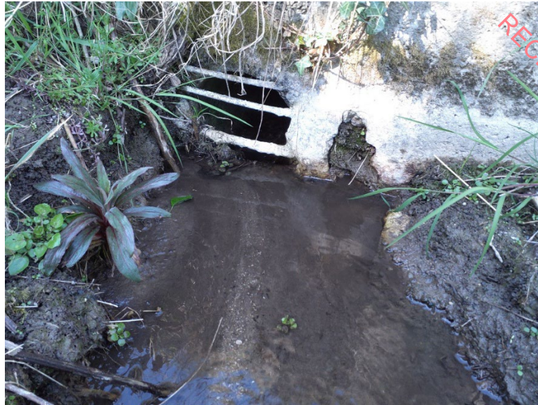
Plate 5-19 Culverted section of the depositing/lowland river habitat along the Coldwater stream
