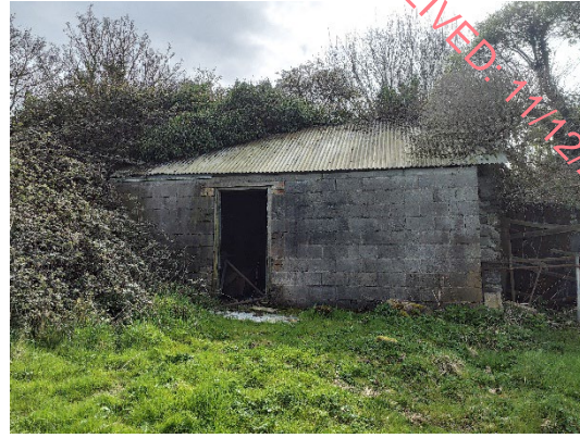
Plate 5-2: Intact building in the southwest of the site
